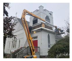
Working on our bell tower – really like the lift. We could use it to replace light bulbs in the sanctuary. They replaced rotted boards and even found evidence of leaks. Screens behind the louvres should keep pushy squirrels at bay.
